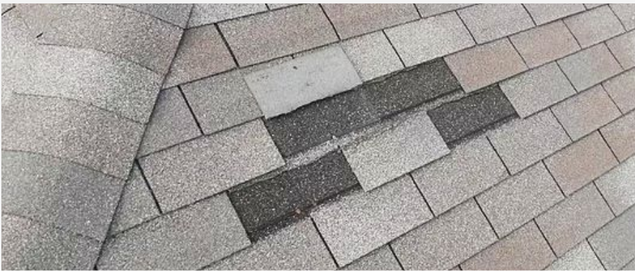
MISSING SHINGLES
